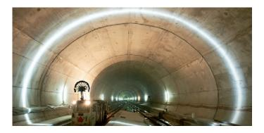
In order to assure tunnel safety, they need to be inspected on a regular basis to detect cracks, scales, spills, or corrosion. In the past, this was mostly done by tunnel personnel using mobile scaffolds. However, this procedure is very time-consuming, labor-intensive and involves the danger of overlooking these troublesome indicators or not recognizing them at an early stage.
